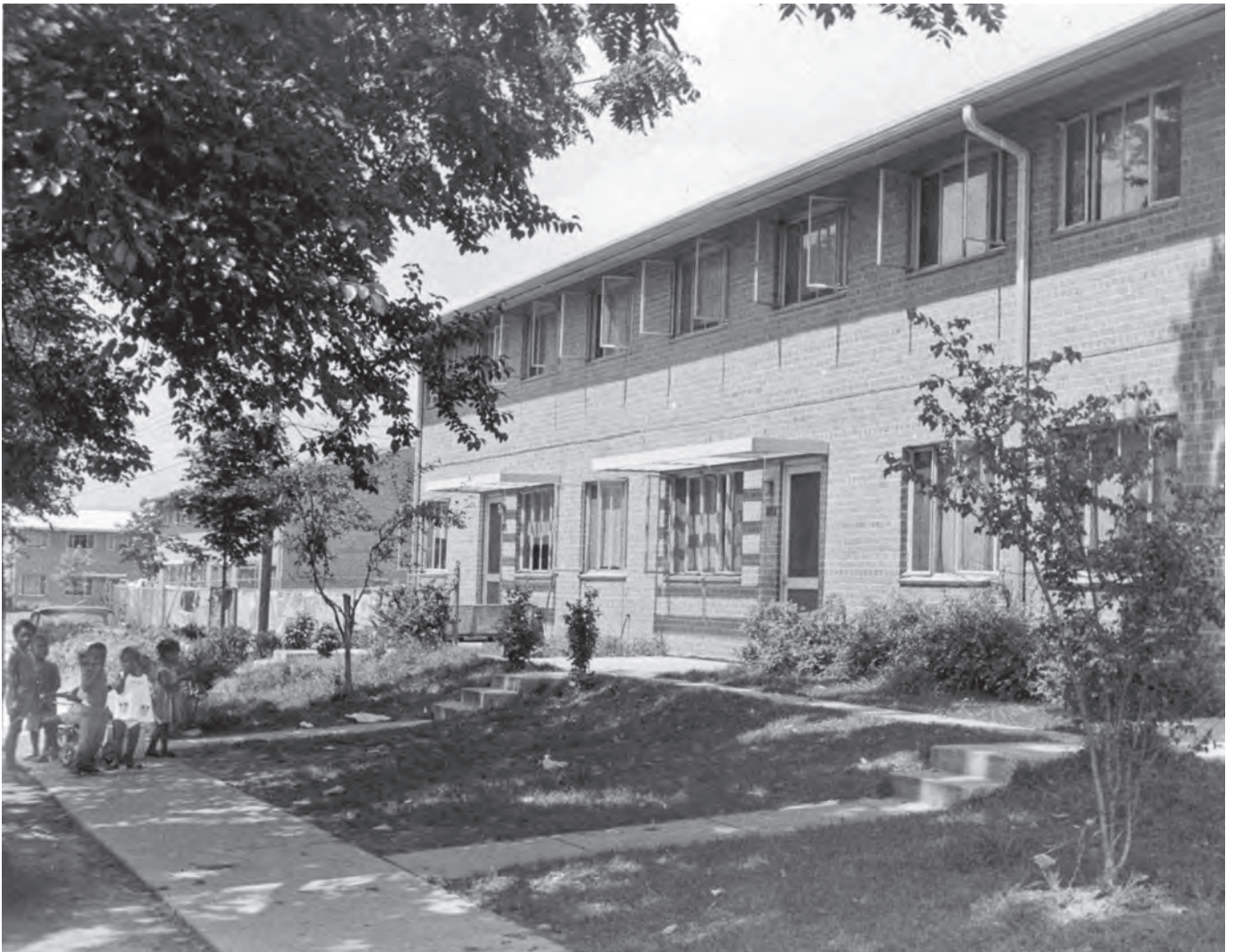
Kenilworth Courts in 1961, two years after it opened. Courtesy, National Capital Housing Authority
